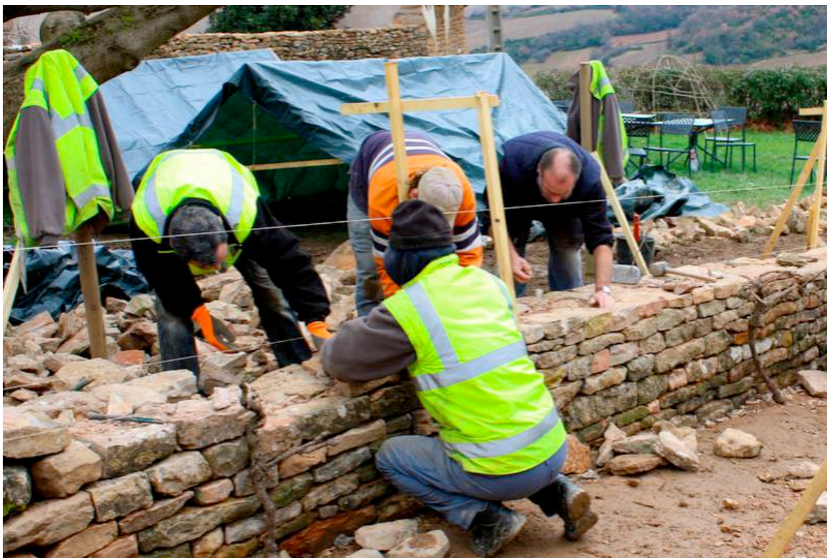
RGSF-4 Solutré-Pouilly-Vergisson, Grand Site de France and its employability team rebuilding a traditional dry stonewall ©RGSF/2013
